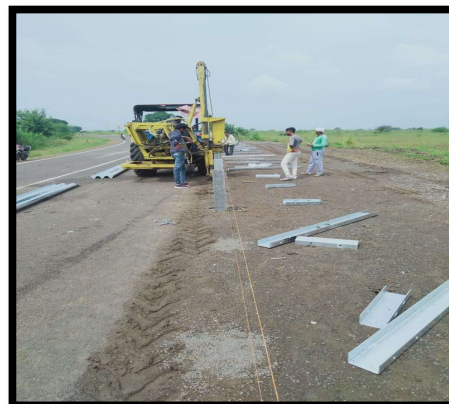
Insertion of end terminal posts as per depth required and drawings.
