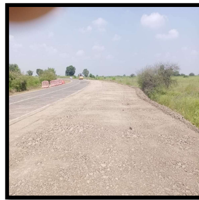
Area Compaction with 10 Ton Roller Compactor
