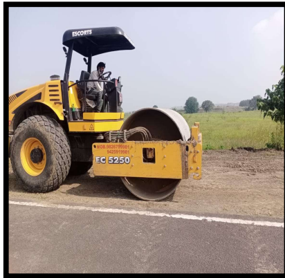
Area Compaction with 10 Ton Roller Compactor
