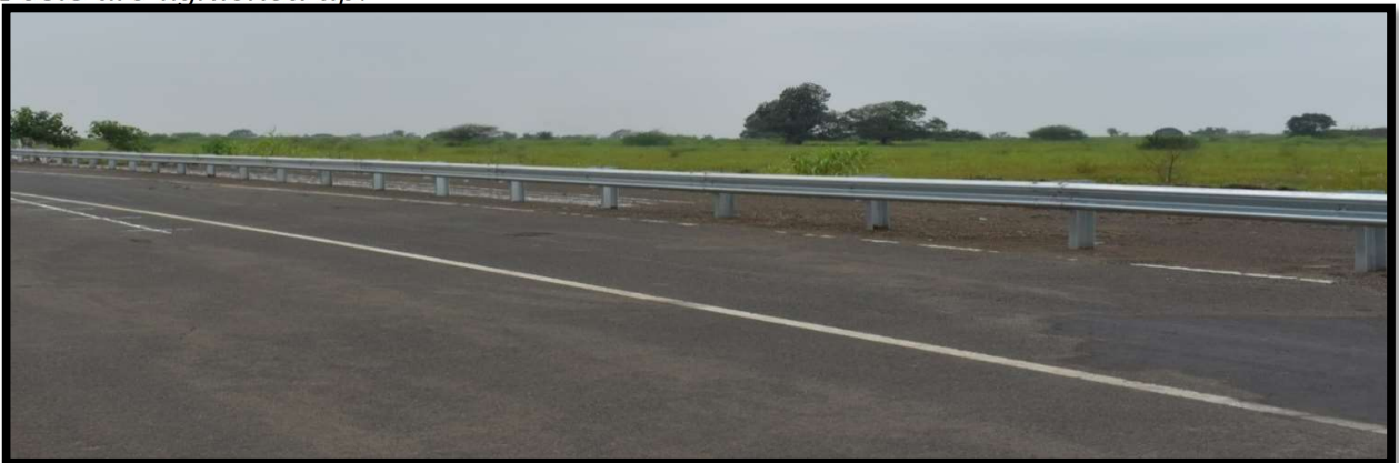
Over all View of Front side beam
