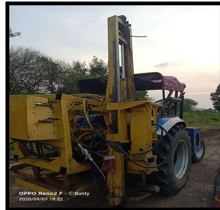
Preparation of Post driving machine as per marking (drawings).
