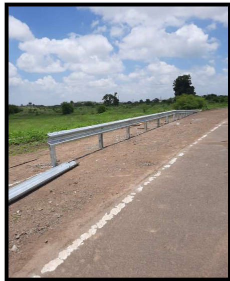
Insertion of remaining post and laying of beams in front of Barrier line
