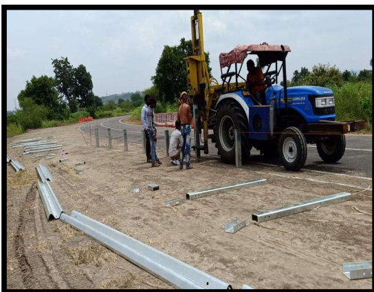
Insertion of end terminal posts as per depth required and drawings.
