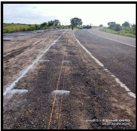
Marking on compacted area from post insertion
